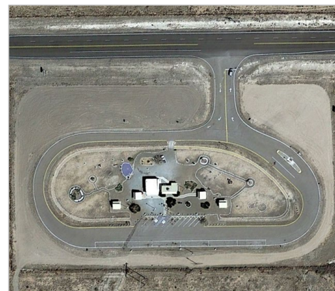
Rest area located at MP 144.6
