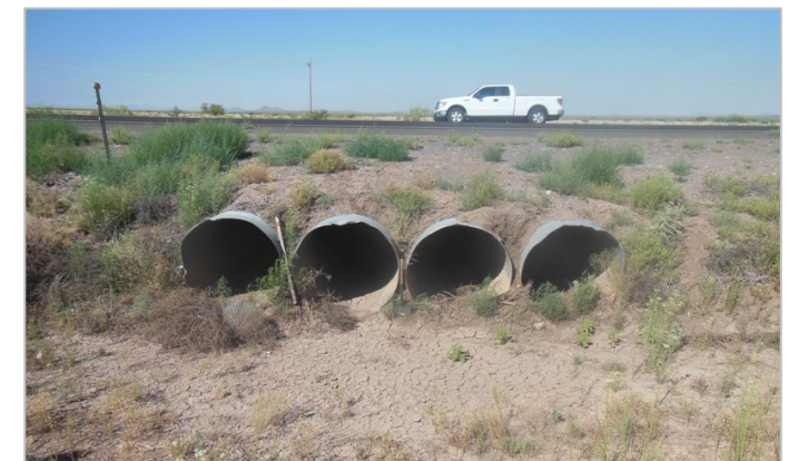
Several box culverts have been extended with adjacent corrugated metal pipes and lack support from surrounding soils.
