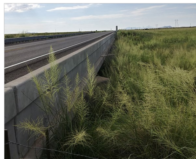
Built in 1970, the US 180 Cold Water Creek Bridge (#7160) is in satisfactory to good condition.
