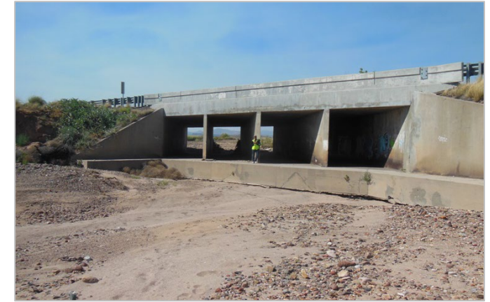
Erosion at the Whitewater Draw culvert at MP 135.15.
