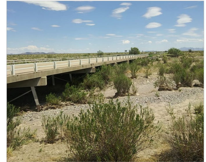
Built in 1980, the Mimbres River Bridge (#8152) is in satisfactory conditions, but overtopping has been reported.
