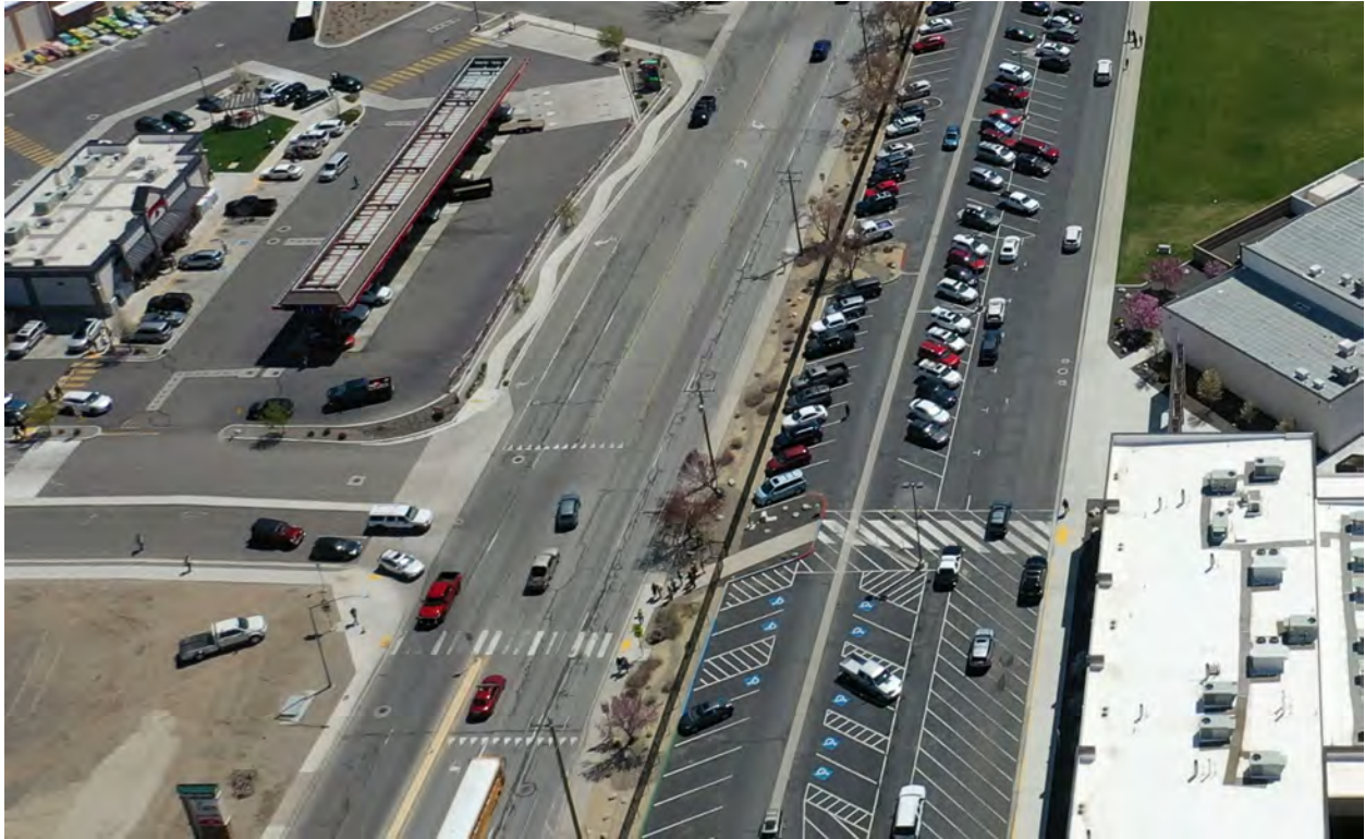
Existing conditions on SR 88 at Douglas High School
