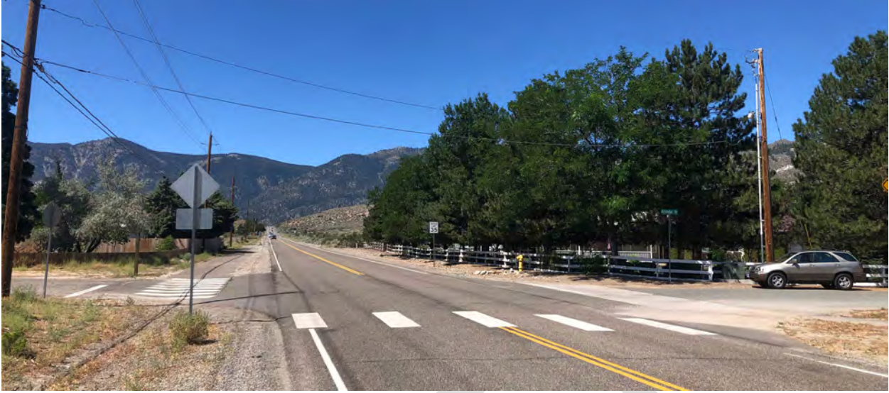
Existing conditions at Jacks Valley Road and Arcadia Drive
