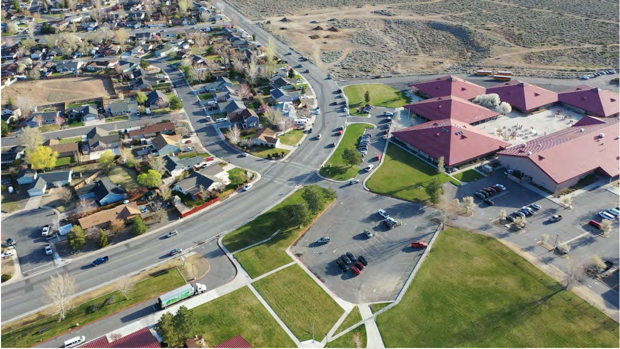
Existing conditions along Long Valley Road
