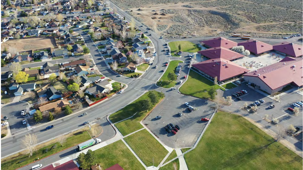
Existing conditions along Long Valley Road
