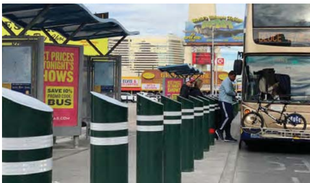
Examples of bollards installed in front of RTC bus stop on Las Vegas Boulevard/Boulder Highway. Image from Google Maps
