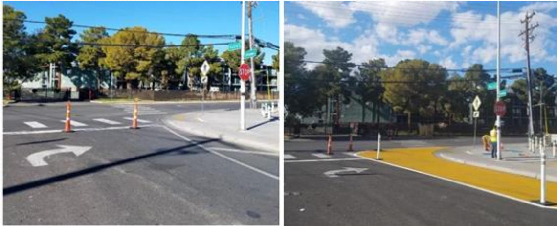
Figure 99: Temporary Sidewalk Extension at Cambridge St. and Katie Ave.
