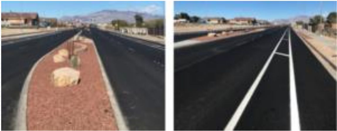
Figure 100: Complete Street Elements on Fort Apache Road in Clark County
