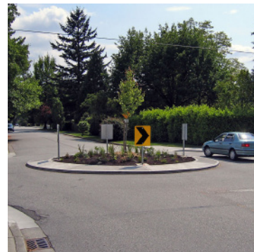
Traffic calming techniques
